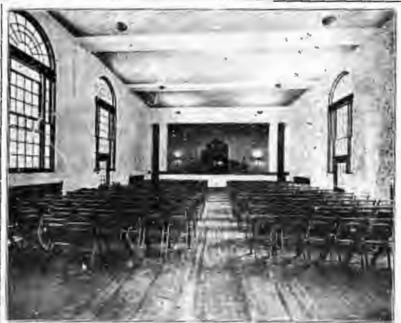
The center prong of the E shaped conservatory is the music auditorium where student recitals and smaller music assemblies can be held. Well lighted, with a deep stage which opens onto the big stage in the Main auditorium, the auditorium will seat 400 persons comfortably.
