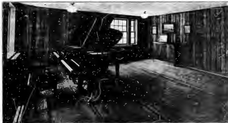
The studio of Dr. Walter Roberts, head of the music department. In the new conservatory is illustrative of the stained paneled walls of the 11 other studios and the 53 practice rooms. Practically sound proof, the many rooms hold varied activities going on at the same time with little interference with each other.
