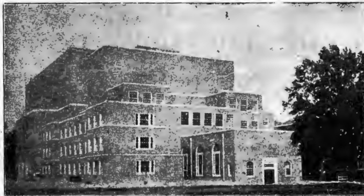
Looking from the rear of the new auditorium, one sees the 3-floor music conservatory part of the structure. With 53 almost sound-proof practice rooms, a music auditorium, two reception rooms, 4 classrooms, a music library, 12 studios, a band and orchestra room, the conservatory is one of the most adequate in the South.
