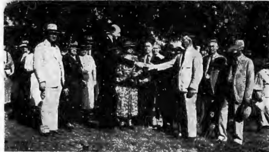
Dr. John McSwain, representing Columbia Presbyterian Theological Seminary, hands a brick out of the original chapel to President Shelton Phelps, symbolic of the handing over of the guardianship of the old building.
