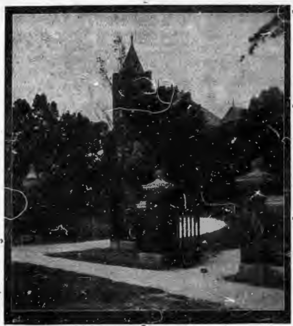
ADMINISTRATION BUILDING OF WINTHROP
