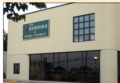
The Bookworm, pictured above, is undergoing renovation to become the new home of the Louise Pettus Archives and Special Collections.
