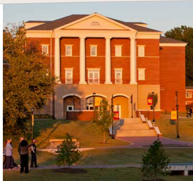
GLENDA PITTMAN AND CHARLES JERRY OWENS HALL Opened in 2007, Owens Hall is Winthrop's newest general-use classroom facility. The 32,200-square-foot building contains 21 classrooms equipped with SMART technology, a computer lab, two conference rooms and a student lounge. Named for Glenda Pittman Owens '59 and her husband, Jerry, the building suffered severe damage from a March 6, 2010, fire and reopened in spring 2011. The space was formerly a parking lot located behind Bancroft Hall.
