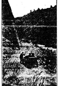
Example of Mountain Road Building in Colorado.
