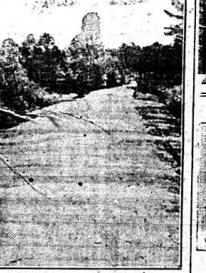
An Improved Southern Road.
