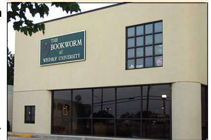
The Bookworm, pictured above, is undergoing renovation to become the new home of the Louise Pettus Archives and Special Collections.
