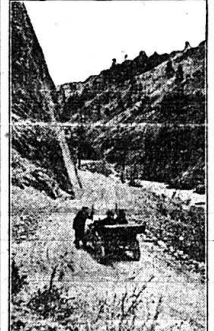
Example of Mountain Road Building in Colorado.
